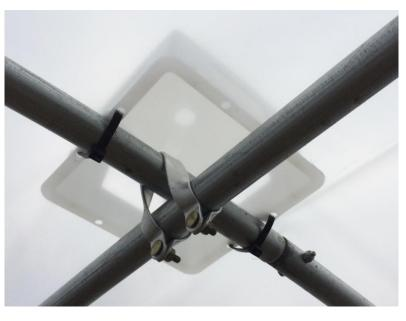
4. Once all blocks are in place, the second layer of plastic can be installed over them. It is important to get this layer as tight as you can before fastening it to your structure. This will help create a more uniform air space as well as help prevent water and snow from accumulating between the spacer blocks.
