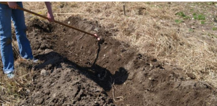
Back-filling the planting trench.
