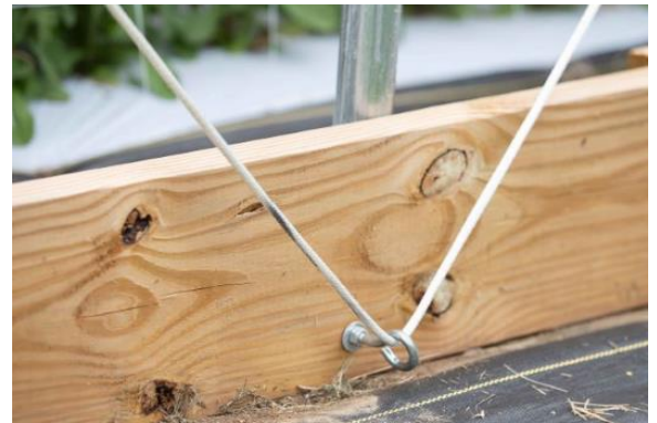
Figure 47: Eyebolts for the bottom of the roll-up sides.
