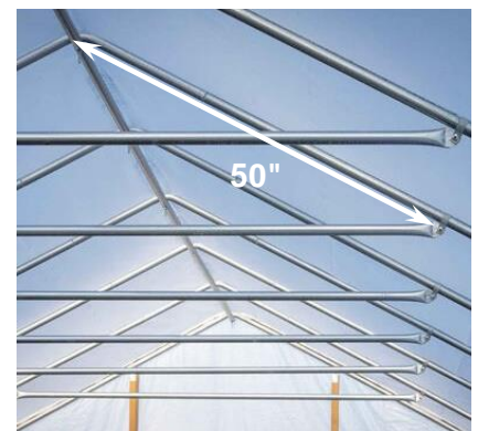
Figure 12: Finished truss installation.
