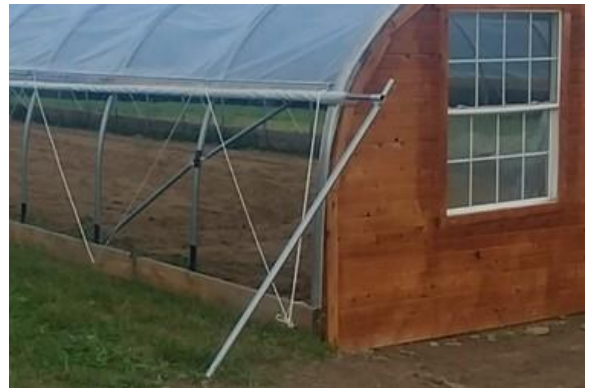
Figure 50: Finished roll-up side with prop bar.
