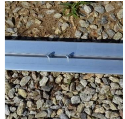
Figure 24: Hex bolts installed in the back side of the channel.
