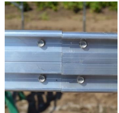
Figure 28: Front view of connector plate installed.
