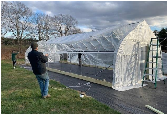
Figure 39: Pulling poly over the tunnel frame.
