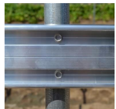
Figure 30: Channel secured to bow with Tek screws.
