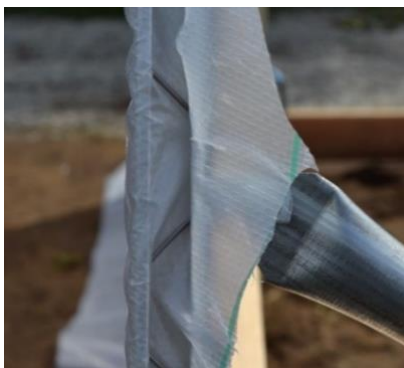
Figure 34: Lock wire installed on end wall bow.
