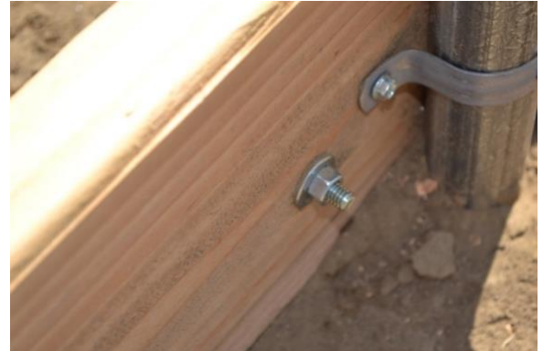
Figure 42: Eyebolt installed from the inside.
