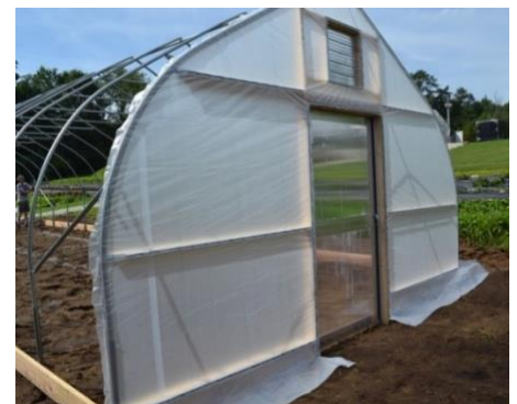
Figure 36: Completed poly installation with excess material removed.
