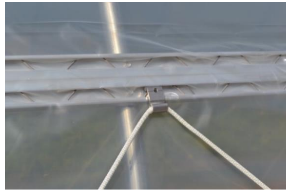
Figure 46: Rope hooks for the top of the roll-up sides.
