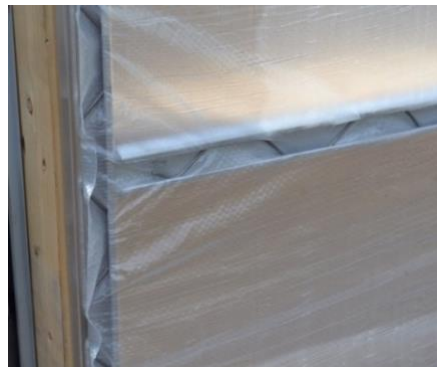
Figure 35: Lock wire installed on vertical and horizontal framing.
