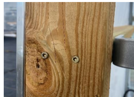
Figure 20: Securing horizontal stud to door frame.
