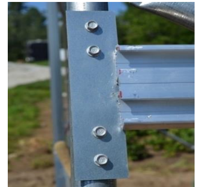
Figure 26: Front view of channel secured to T-plate.
