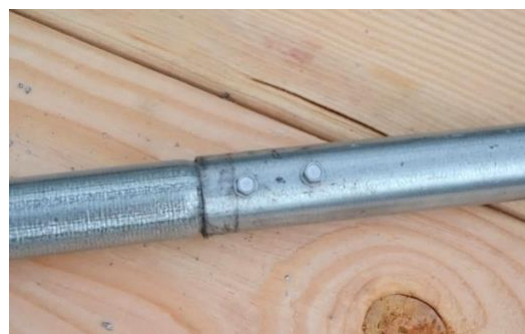
Figure 6: Tek screws securing bow assembly.
