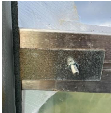
Figure 25: Back view of channel secured to T-plate.
