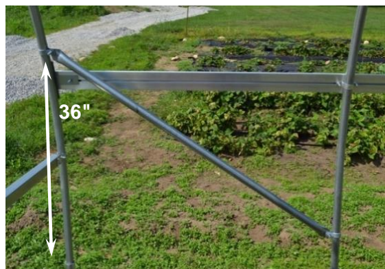
Figure 13: Wind brace attached 36" above the top of the ground post.
