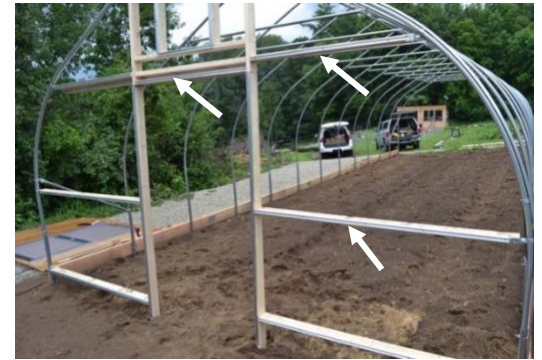
Figure 32: Channel installed on end wall framing.
