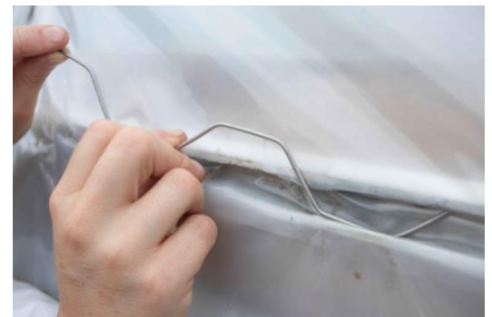
Figure 33: Installing wire lock into channel.
