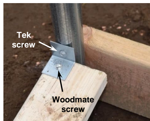
Figure 22: Securing bottom 2 x 4 to end wall frame.
