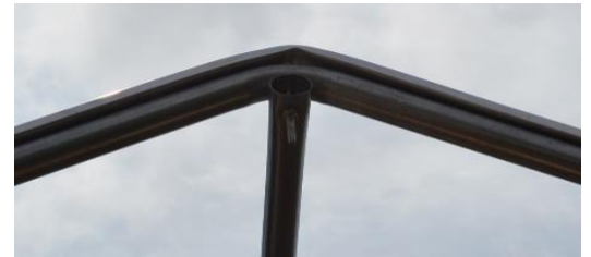
Figure 31: Channel attached to bow peak
