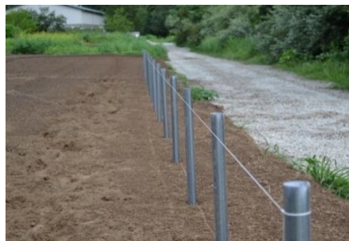
Figure 4: Level ground posts and mason line.
