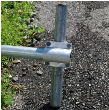
Figure 48: U-bracket for T-handle.
