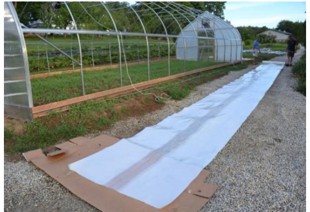
Figure 37: Roll out poly along tunnel.
