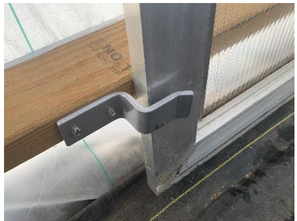
Figure 11: Z-stop installed.
