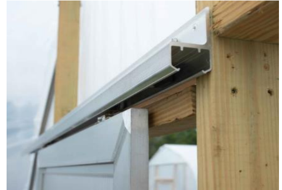
Figure 1: Door track installed.
