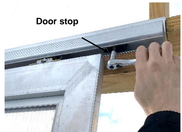
Figure 9: Door stop for closed position.
