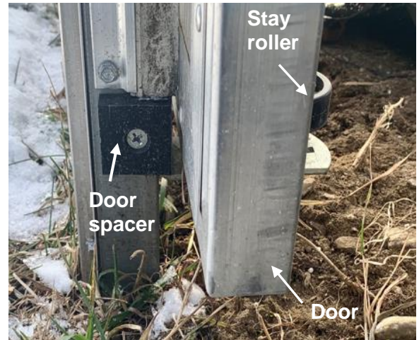
Figure 8: Door spacer opposite the stay roller.
