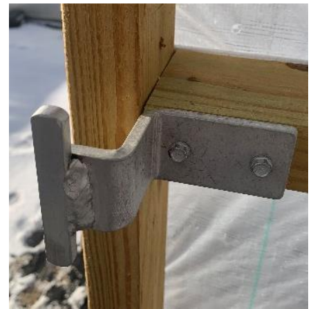
Figure 12: Z-catch installed.
