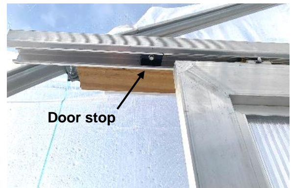
Figure 10: Door stop for open position.
