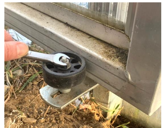
Figure 7: Adjusting the stay roller.
