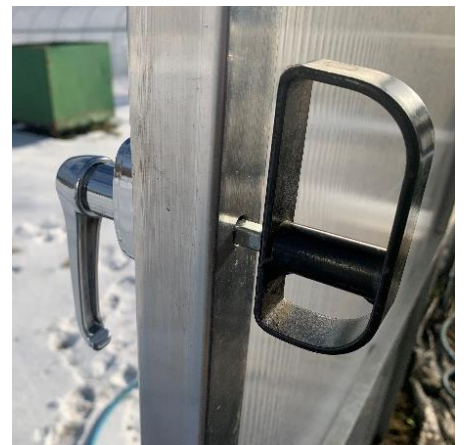
Figure 13: Handle assembly installed.
