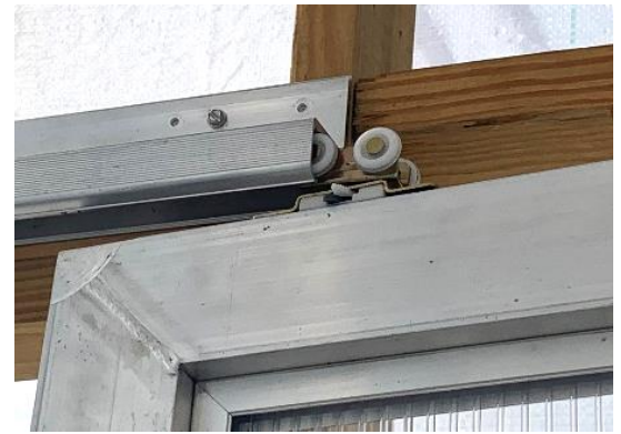
Figure 4: Mounting the door into the track.
