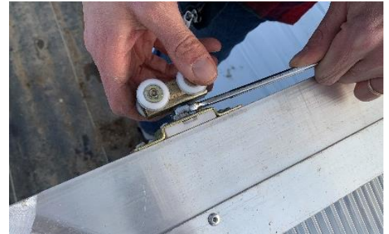
Figure 5: Adjust the height of the door.
