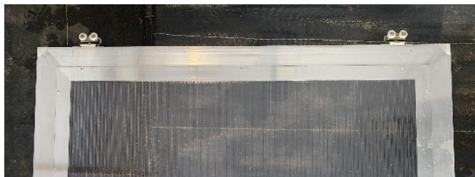
Figure 2: Door rollers installed.
