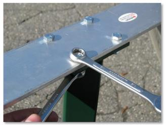
**STEP 4:** Using the two ½" wrenches, secure the mounting plate with the 4 screws, washers, and hex nuts provided as shown above.
