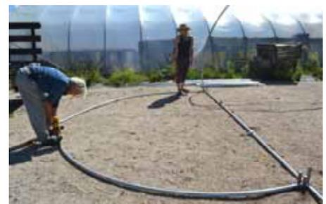
8. Slip a 1-3/8" brace band over the end of each end of the bow and slide them up, towards to the peak section.
