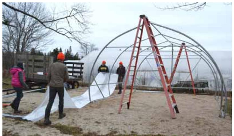
6. With a couple people on the ladders, pass the pre-cut sheet of plastic up and over the tunnel module frame.
