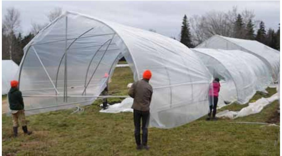
*Moving the Modular Cathedral into place in November over crops started in fall under Quick Hoops low tunnels*
