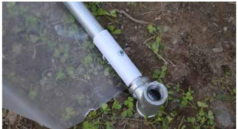
iii. Lay the EMT assembly on the loose plastic at the bottom of one side of a tunnel module. Wrap it around the EMT evenly and secure in place with Snap Clamps every foot or so. Adjust Snap Clamps as necessary, removing any wrinkles in the plastic and ensuring that the EMT is parallel to the horizontal channel.
