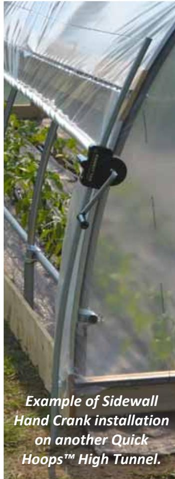
*Example of Sidewall Hand Crank installation on another Quick Hoops™ High Tunnel.*
