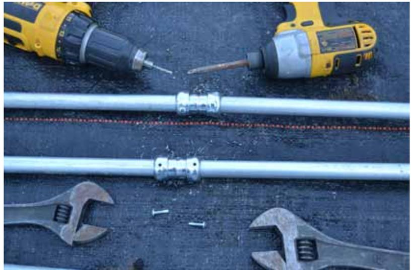
ii. Attach the T-fitting to one end of this now 16.5 ft. piece of EMT. Fully insert the EMT into it. You may need to 'thread' it on. Drive a tek screw through it and into the EMT inside it to keep it from slipping.
