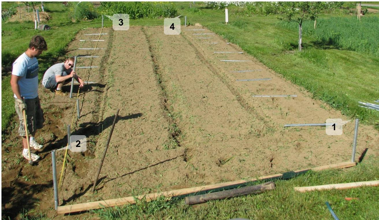
4. **If you choose to forgo weed barrier, proceed as follows:** Set the 4 corner ground posts first (refer to the diagram, on page 8 for this part of the procedure).
