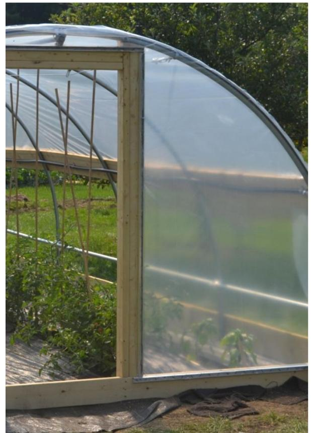
**6. Skinning the Main Portion of the Tunnel:** This process is best done with little or no wind. If possible, postpone this portion of the procedure if the weather is not cooperative.
