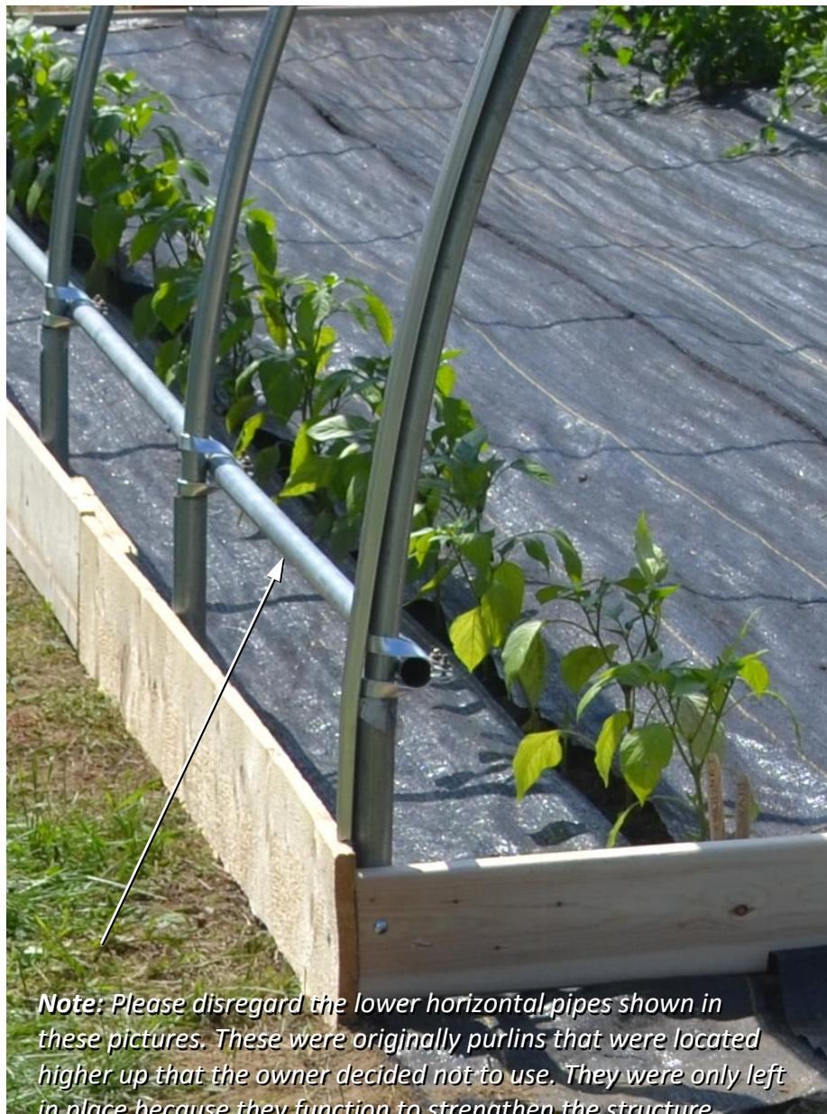
*Note: Please disregard the lower horizontal pipes shown in these pictures. These were originally purlins that were located higher up that the owner decided not to use. They were only left in place because they function to strengthen the structure.*
