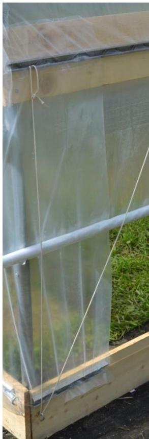
On the side of the tunnel, pull the bottom end of the plastic tight and poly latch wire a 2-foot section into the end of the hipboard and the small section of poly latch wire channel on the side baseboard below it.
