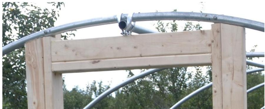
Hold a 2X4 horizontally across the inside of the top of the doorway. Place one edge of it against the left inner door frame board and behind the right door frame boards. Using the right door frame board as a guide, make a mark on the 2X4 on the inside edge of the frame. Cut 2 pieces of 2X4 to this length.
