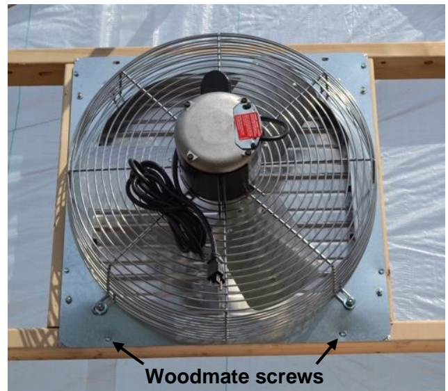
Figure 1: Exhaust shutter fan installed.
