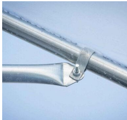
Figure 1: Brace band securing truss to Bobcat frame.
