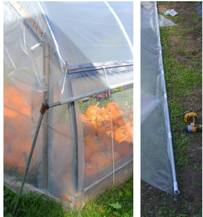
b. **Sidewall Hand Crank Roll-ups:** This design uses ¾-inch EMT conduit, ¾-inch EMT compression fittings, Snap Clamps, #8 x ¾-inch Phillips-head self-drilling tek screws, and Sidewall Hand Crank.
