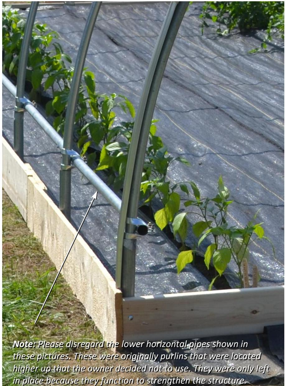
2. **Hipboards:** These provide some bracing for the tunnel and a convenient place to mount poly latch wire channel. They are typically made out of 1-inch X 6-inch or 2-inch X 6-inch board. In this picture, we used the same 1-inch X 8-inch ledger board for hipboards on this smaller tunnel. On the longer tunnels at our farm, we used 1-inch X 6-inch boards.
