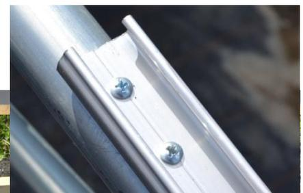
hipboard. Center it vertically and clamp it in place. Using #8 X ½-inch Phillips-head self-drilling tech screws, secure it in place. Phillips head screws are used to prevent damage to the plastic. Install screws every foot or so. Butt a second piece up to the end of the first and secure in place. Repeat down both sides of the tunnel. Use a hack saw or reciprocating saw to cut the final pieces to length prior to attaching.
