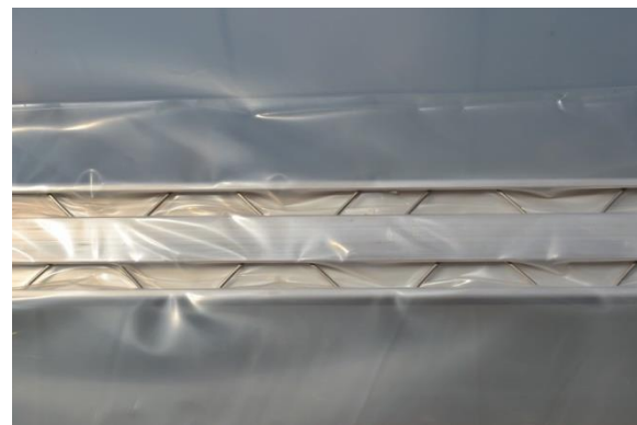
Figure 41: Wire lock installed in both side wall channels.
