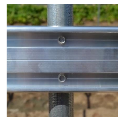
Figure 29: Channel secured to bow with Tek screws.
