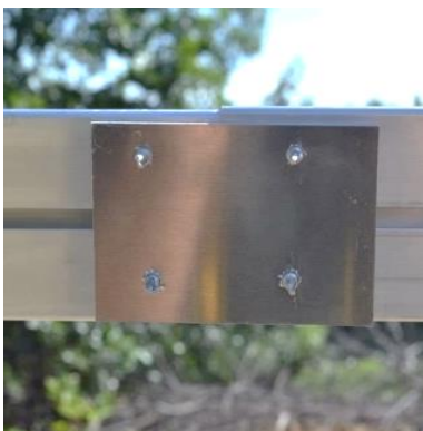
Figure 28: Back view of connector plate installed.
