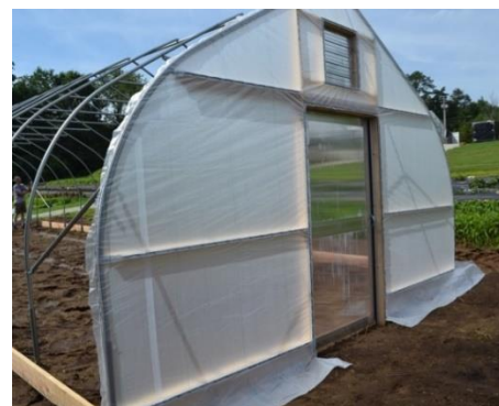
Figure 35: Completed poly installation with excess material removed.
