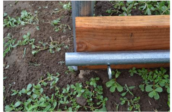
Figure 44: Pipe extending 1" beyond the outside edge.
