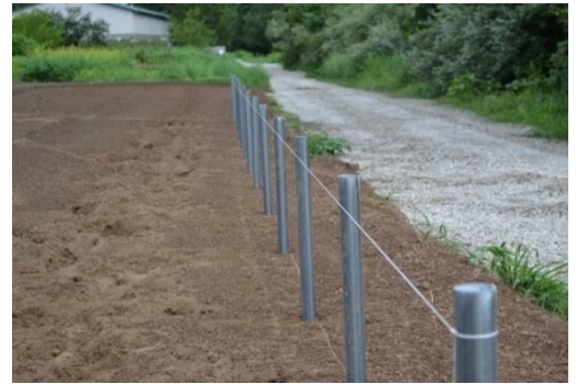
Figure 4: Level ground posts and mason line.
