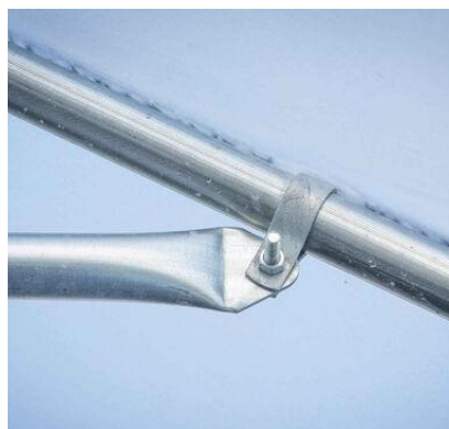
Figure 11: Brace band securing trusses to Bobcat frame.
