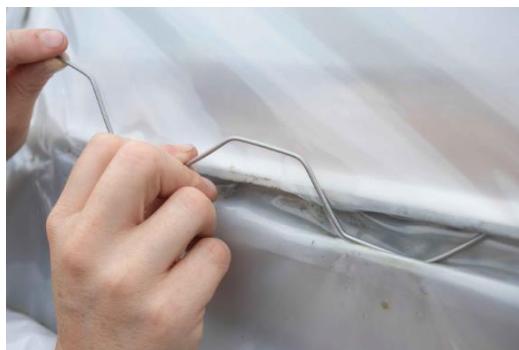
Figure 32: Installing wire lock into channel.
