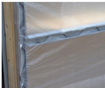
Figure 34: Lock wire installed on vertical and horizontal framing.
