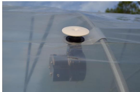
Figure 37: Blower installed in the first poly layer.
