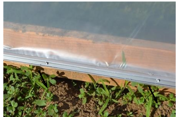
Figure 46: Tek screws securing curtain cap to the roll-up side pipe.
