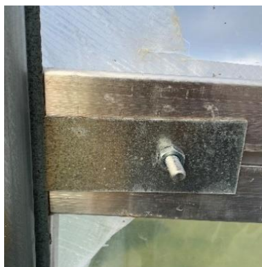
Figure 24: Back view of channel secured to T-plate.
