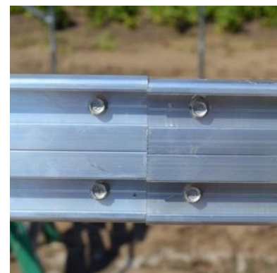
Figure 27: Front view of connector plate installed.
