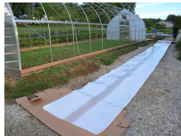
Figure 38: Roll out poly along tunnel.
