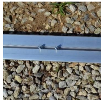
Figure 23: Hex bolts installed in the back side of the channel.
