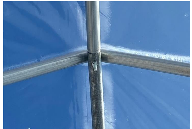
Figure 10: Ridge purlin secured to the bow peak.
