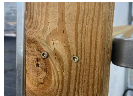
Figure 19: Securing horizontal stud to door frame.
