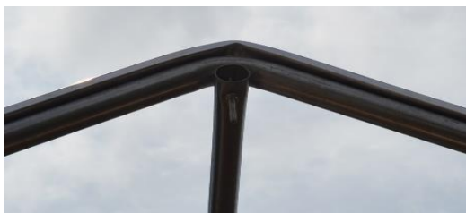
Figure 30: Channel attached to bow peak.
