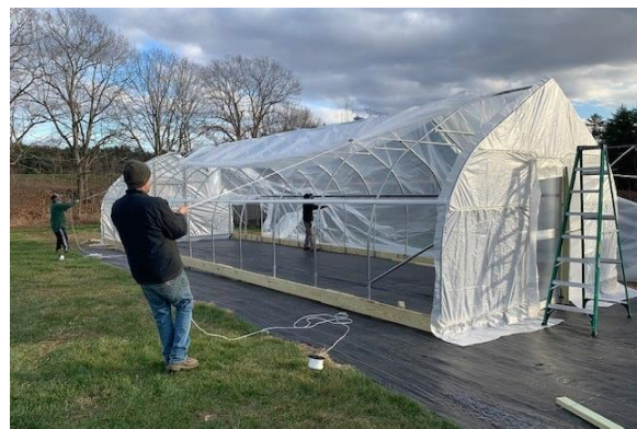
Figure 40: Pulling poly over the tunnel frame.
