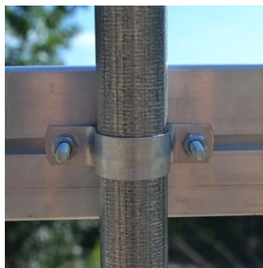
Figure 26: Securing channel to the bow with a 2-hole pipe strap.
