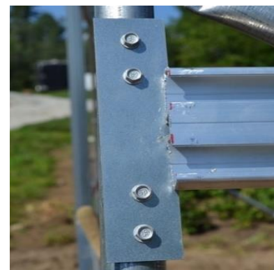
Figure 25: Front view of channel secured to T-plate.
