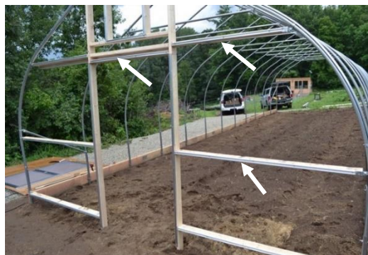
Figure 31: Channel installed on end wall framing.
