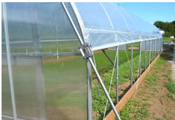
Figure 51: Gear box on the hanging guide pipe.
