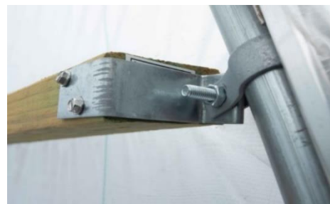
Figure 18: Connecting a 2 x 4 to the frame with an end wall bracket and brace band.
