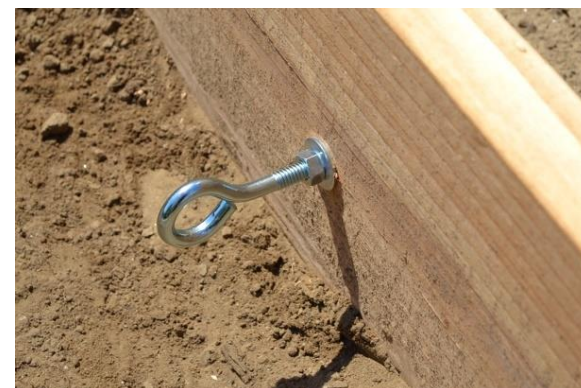
Figure 42: Eyebolt view from outside the tunnel.
