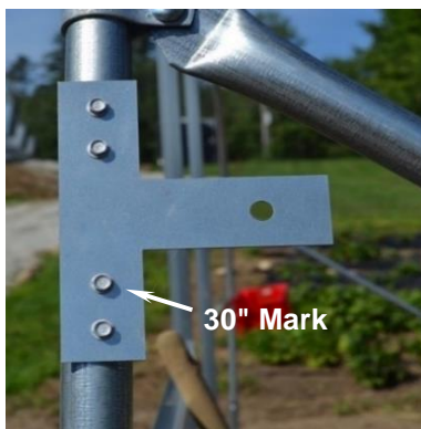
Figure 22: Marks the bottom of the double wire lock channel.
