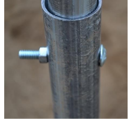
Figure 9: Carriage bolt properly installed.
