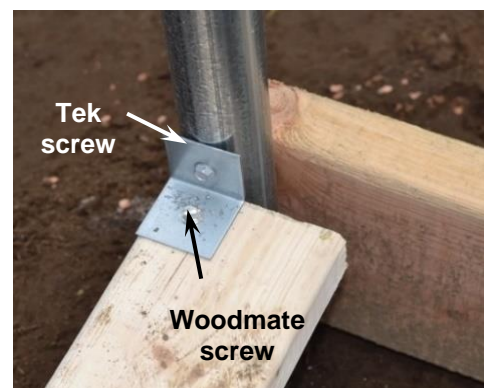
Figure 21: Securing bottom 2 x 4 to end wall frame.
