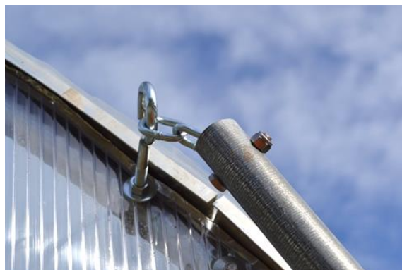
Figure 50: Hardware for mounting the guide pipe.
