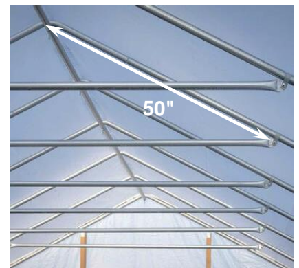
Figure 12: Finished truss installation.
