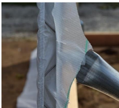
Figure 33: Lock wire installed on end wall bow.
