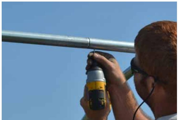
3. **Angle Ties:** at this point, angle ties must be installed so that all successive bows are vertical and plumb. Slip a 1-3/8" brace band over one of the side hoops of one of the end wall bows, two 1-3/8" brace bands over the next bow, and one 1-5/8" brace band over the third ground post.
