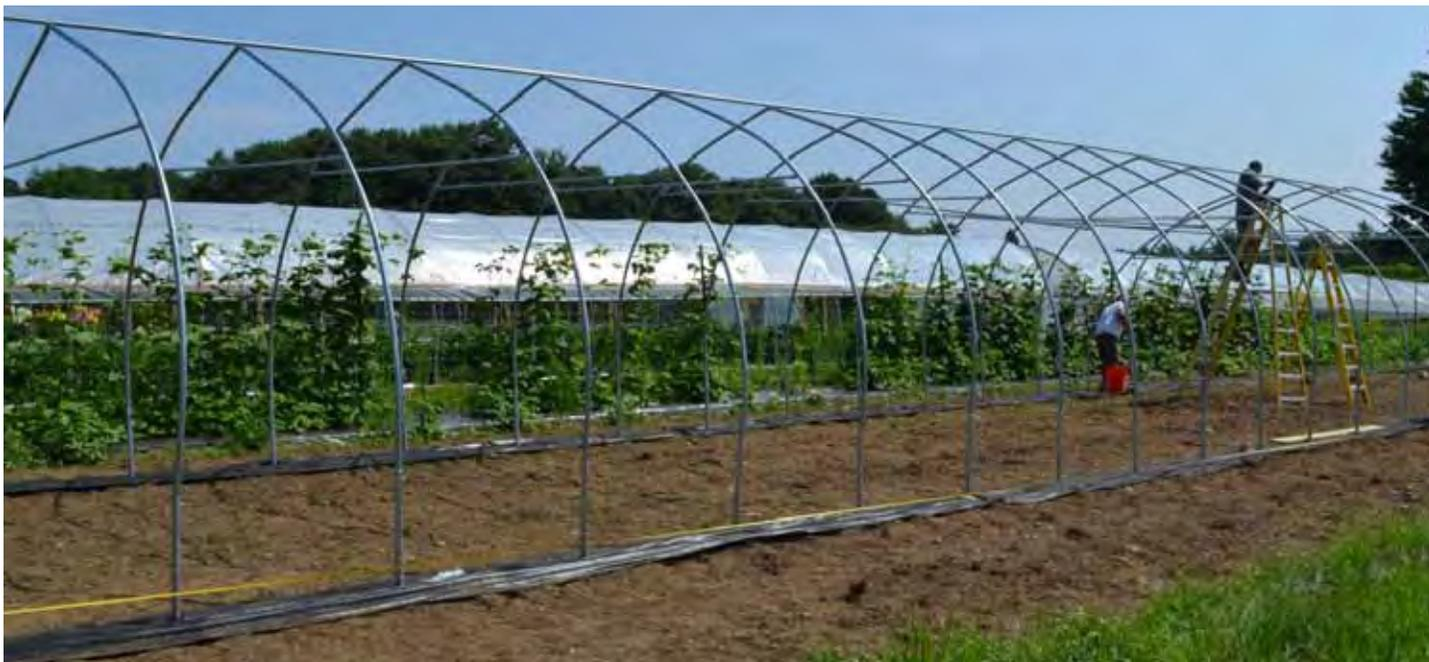
4. **Ridge Pole (continued):** continue adding sections of ridge pole and securing to the peak connector of each bow every four feet as before until you reach the end of the tunnel and have a section of ridge pole protruding out over the opposite end wall.
