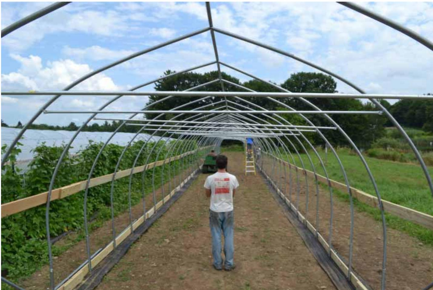
8. **Collar Tie Adjustment:** at this point, the collar ties must be adjusted so that they are somewhat level (with respect to the tunnel) and secured in place. These are not really meant to be truly level because the tunnel may not necessarily be built on level ground. They will simply be adjusted for evenness and aesthetics and secured in place.
