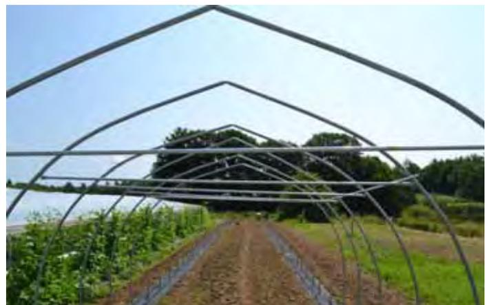
2. **Ridge Pole:** pre-drill a 5/16" hole through the non-swaged end of a piece of 1-3/8" top rail for chain link fence at about 9/16" from the end. Drill through both walls. This will serve as the first piece of ridge pole. Note: if you intend to install scissor doors on this end of the tunnel, you will need about 4" of ridge pole protruding over the end of the tunnel; in that case, drill the hole 4-9/16" from the end of the top-rail.
