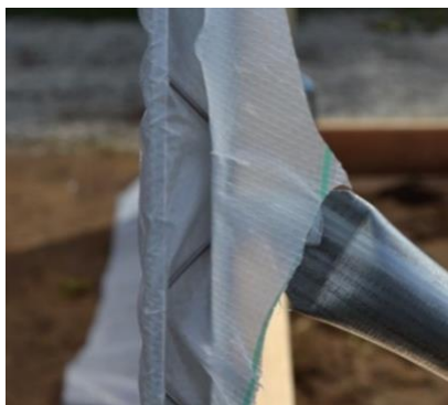
Figure 34: Lock wire installed on end wall bow.
