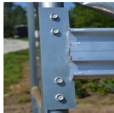
Figure 26: Front view of channel secured to T-plate.
