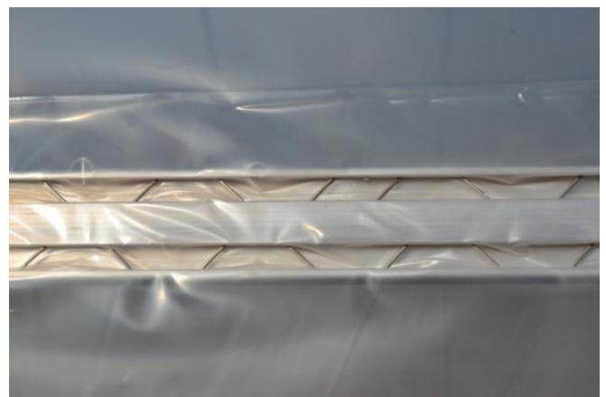
Figure 40: Wire lock installed in both side wall channels.
