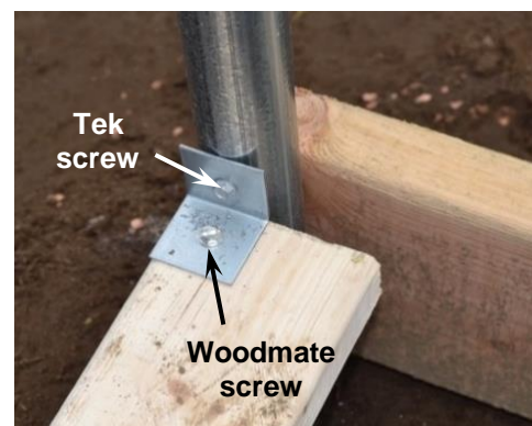
Figure 22: Securing bottom 2 x 4 to end wall frame.
