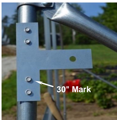
Figure 23: Marks the bottom of the double wire lock channel.
