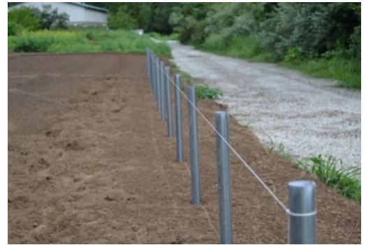
Figure 4: Level ground posts and mason line.
