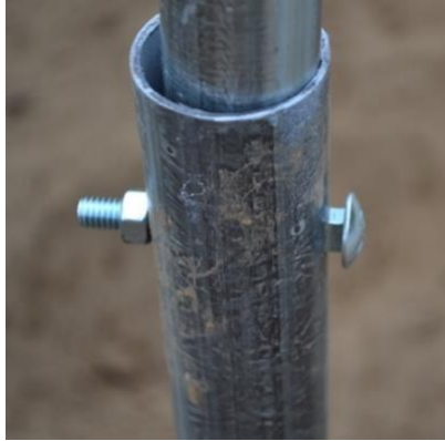
Figure 8: Carriage bolt and hex nut.
