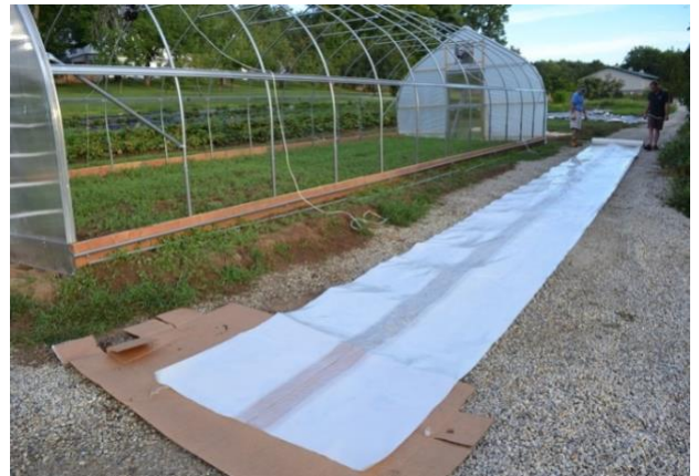
Figure 37: Roll out poly along tunnel.
