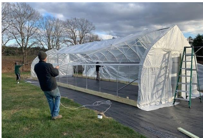
Figure 39: Pulling poly over the tunnel frame.
