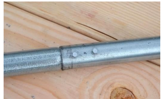
Figure 6: Tek screws securing bow assembly.
