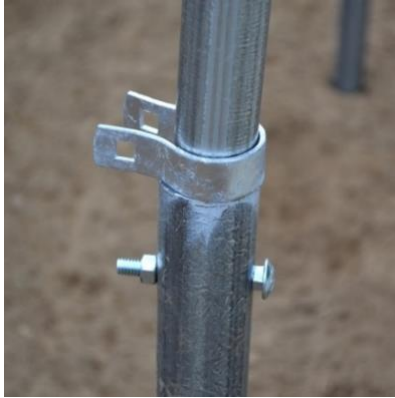
Figure 7: Brace band on end bow for wind bracing, trusses, and framing.
