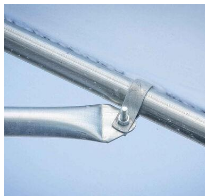
Figure 11: Brace band securing trusses to Bobcat frame.
