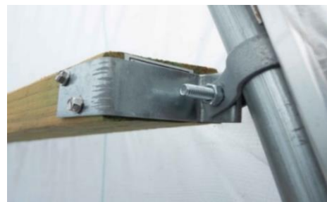
Figure 19: Connecting a 2 x 4 to the frame with an end wall bracket and brace band.
