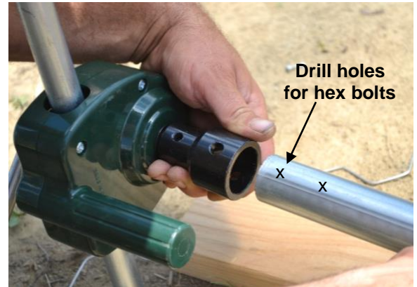
Figure 48: Installing the #7033 Sidewall Hand Crank.
