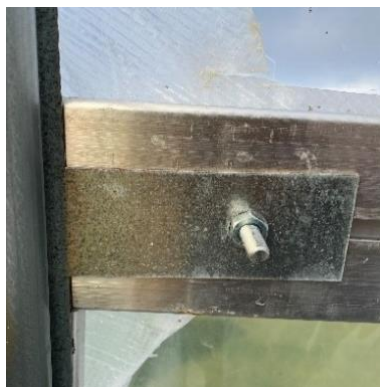
Figure 25: Back view of channel secured to T-plate.
