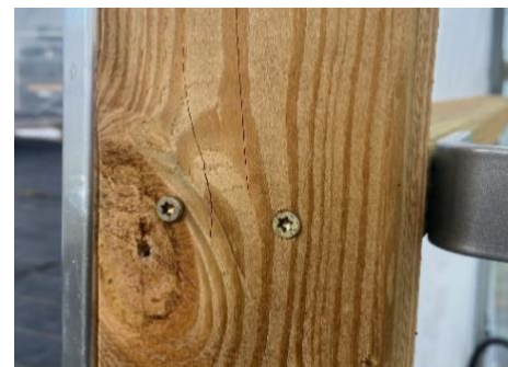
Figure 20: Securing horizontal stud to door frame.
