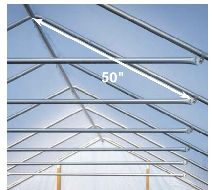
Figure 12: Finished truss installation.
