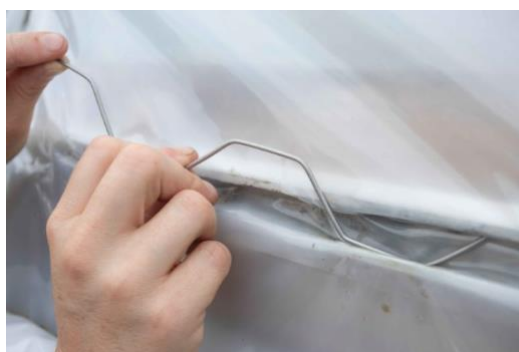
Figure 33: Installing wire lock into channel.
