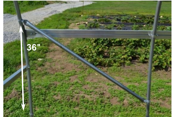
Figure 13: Wind brace attached 36" above the top of the ground post.
