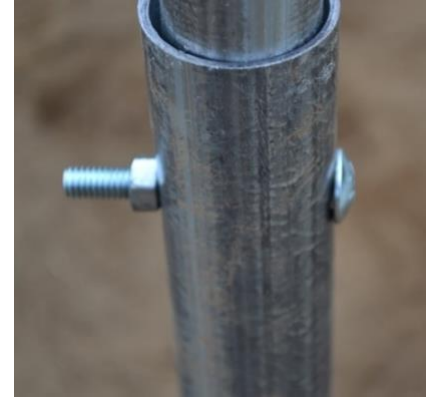
Figure 9: Carriage bolt properly installed.
