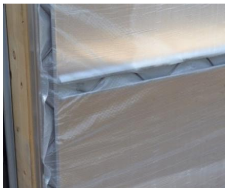
Figure 35: Lock wire installed on vertical and horizontal framing.
