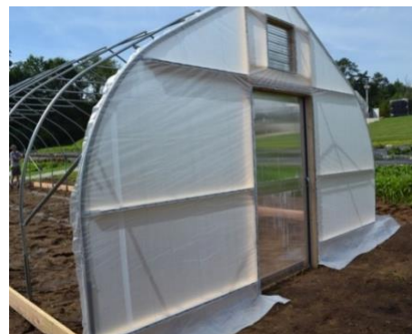
Figure 36: Completed poly installation with excess material removed.
