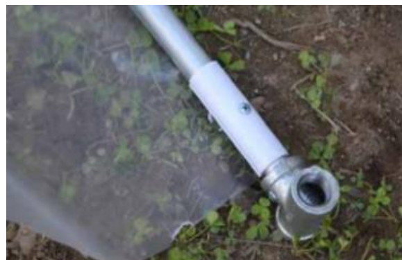
Figure 45: T-fitting and poly film installed on roll-up side.
