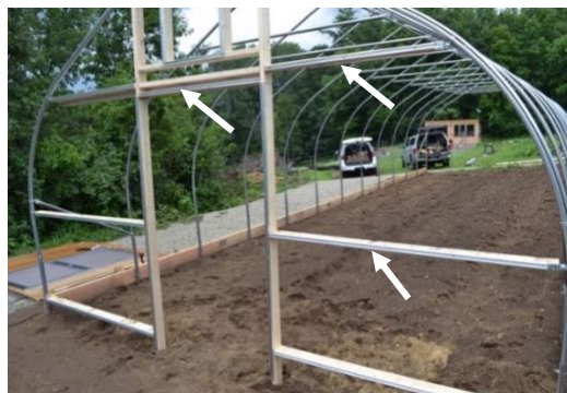
Figure 32: Channel installed on end wall framing.
