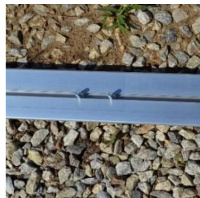
Figure 24: Hex bolts installed in the back side of the channel.
