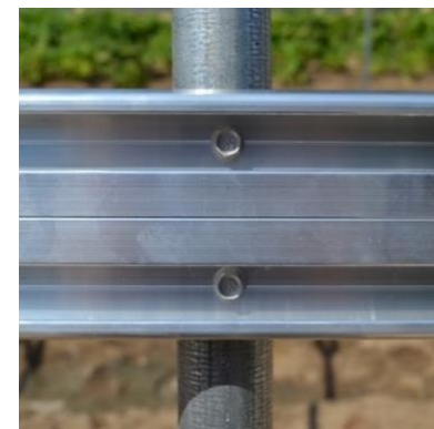
Figure 30: Channel secured to bow with Tek screws.
