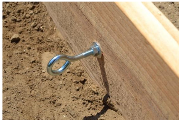
Figure 41: Eyebolt view from outside the tunnel.
