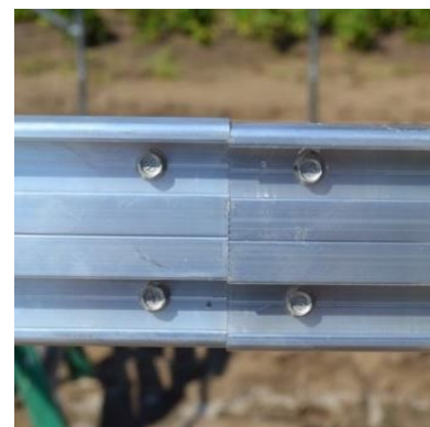
Figure 28: Front view of connector plate installed.
