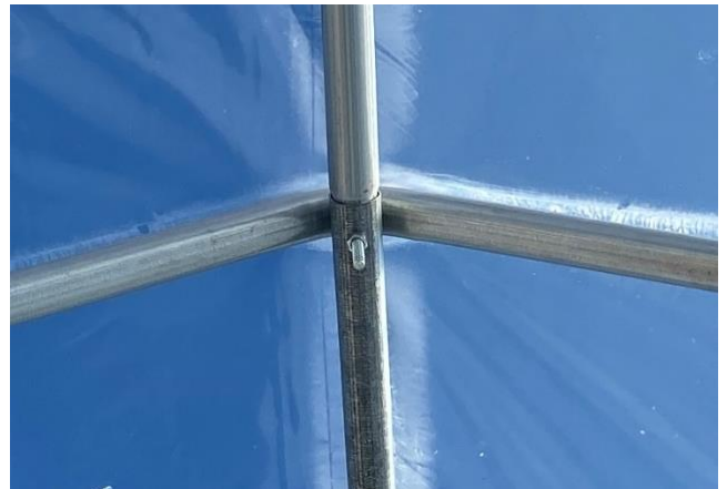
Figure 10: Ridge purlin secured to the bow peak.
