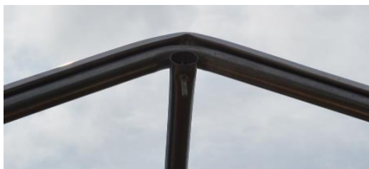
Figure 31: Channel attached to bow peak
