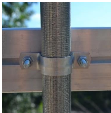
Figure 27: Securing channel to the bow with a 2-hole pipe strap.
